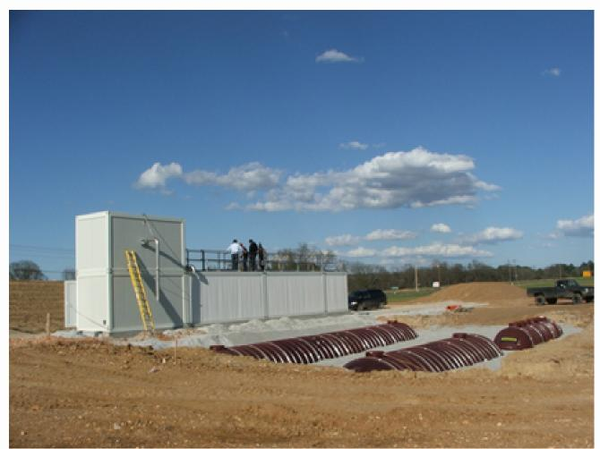
A system like the one above could serve 400 homes and only require around 3 hours per week to operate. The only cost associated with this system is electricity cost of around \$800 per month. The current market for wastewater monthly utility fees is around \$65/home.
